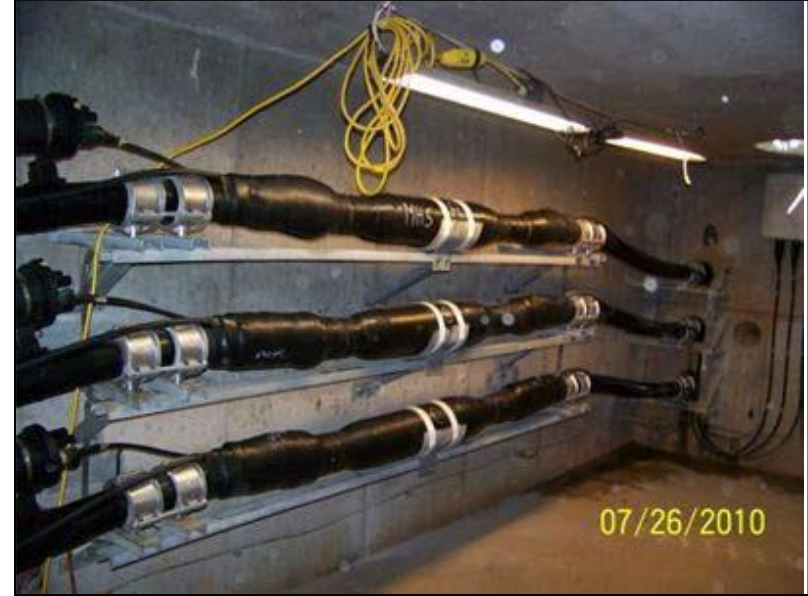
Cable Splicing within vault
