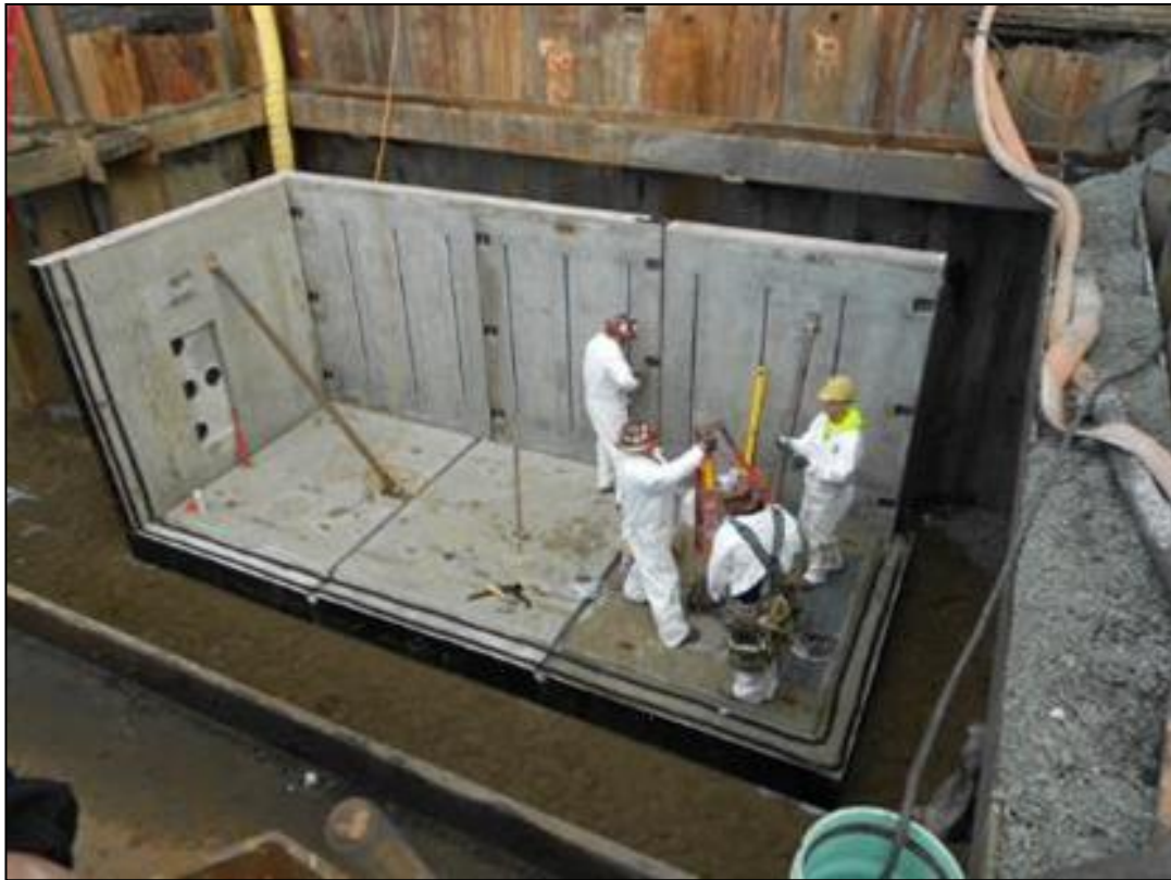
Cable splice vault
