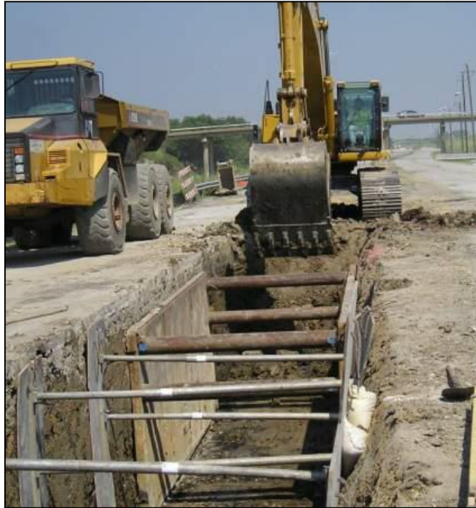
Cable Duct Bank Excavation
