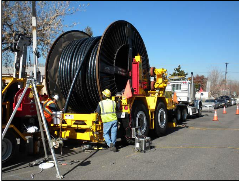
Cable Installation Approximately 2,000 ft cable lengths
